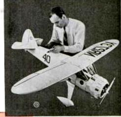
After covering fuselage and wings, the parts are sprayed with water, allowed to dry theroughly, then given two costs of airplane wing dope. When dry this is followed with a cost of white longuer applied with a comet's hair break
